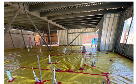
Above: Prep for new slab to be poured. Yellow material is under-slab vapor barrier.
